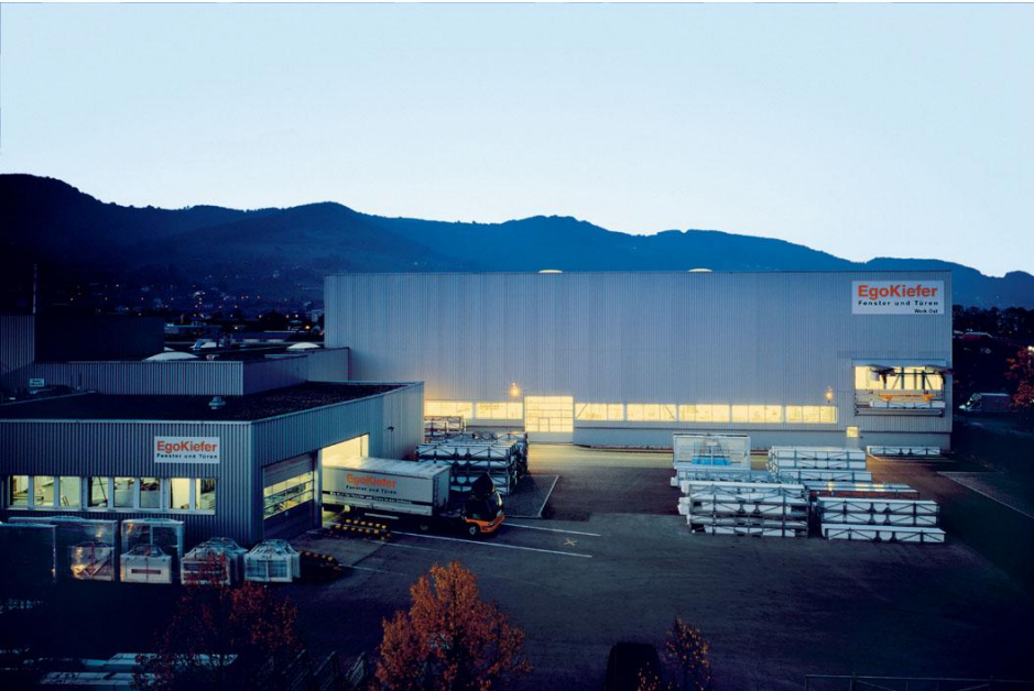
Usine Altstätten Ost
